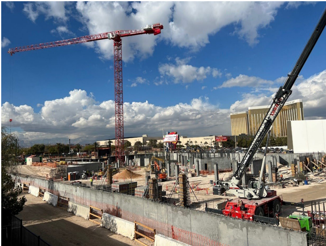
Figure 2 – Project site on December 7, 2022
